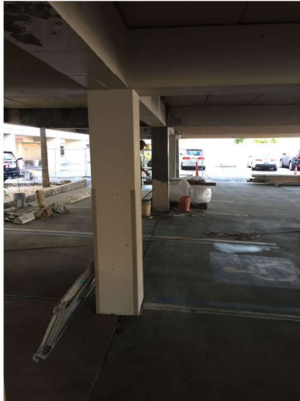
Picture 1: In-progress stucco application
